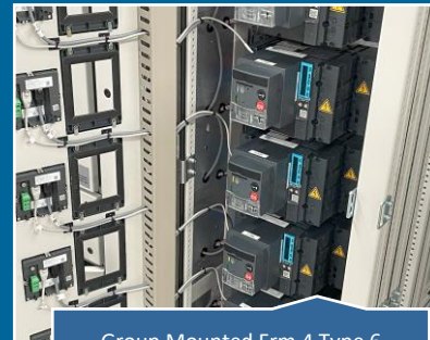
Group Mounted Form 4 Type 6 switchboard with automatic load shedding
