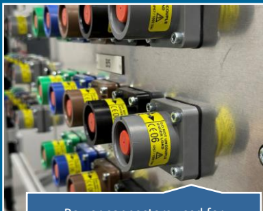
Power connectors used for connection of a temporary generator or load bank
