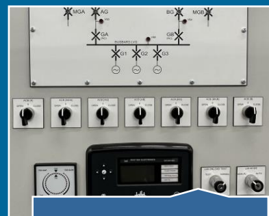
Power Management with integrated Deep Sea controller
