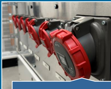
Appliance outlets integrated into a switchboard
