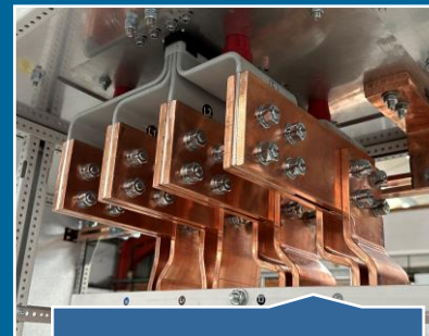
Internal copper connections onto busbar flange.
