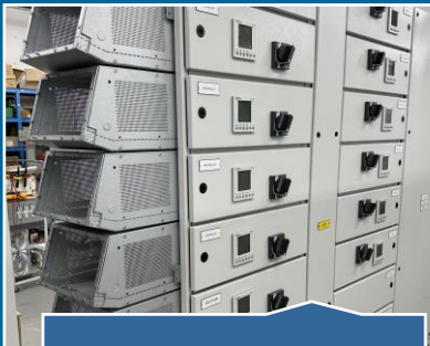
Form 4 Type 6 cable boxes on a front access switchboard
