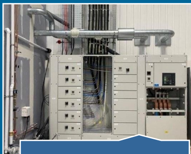
Switchboard being installed
