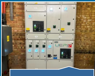
Vertically oriented MCCB compartments
