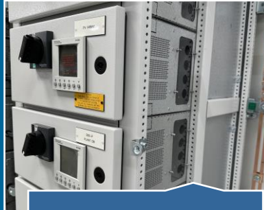
Small MCCB compartments with metering - Form 4 Type 2
